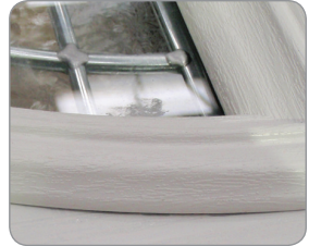
Boss correct way around - low lip on glass
