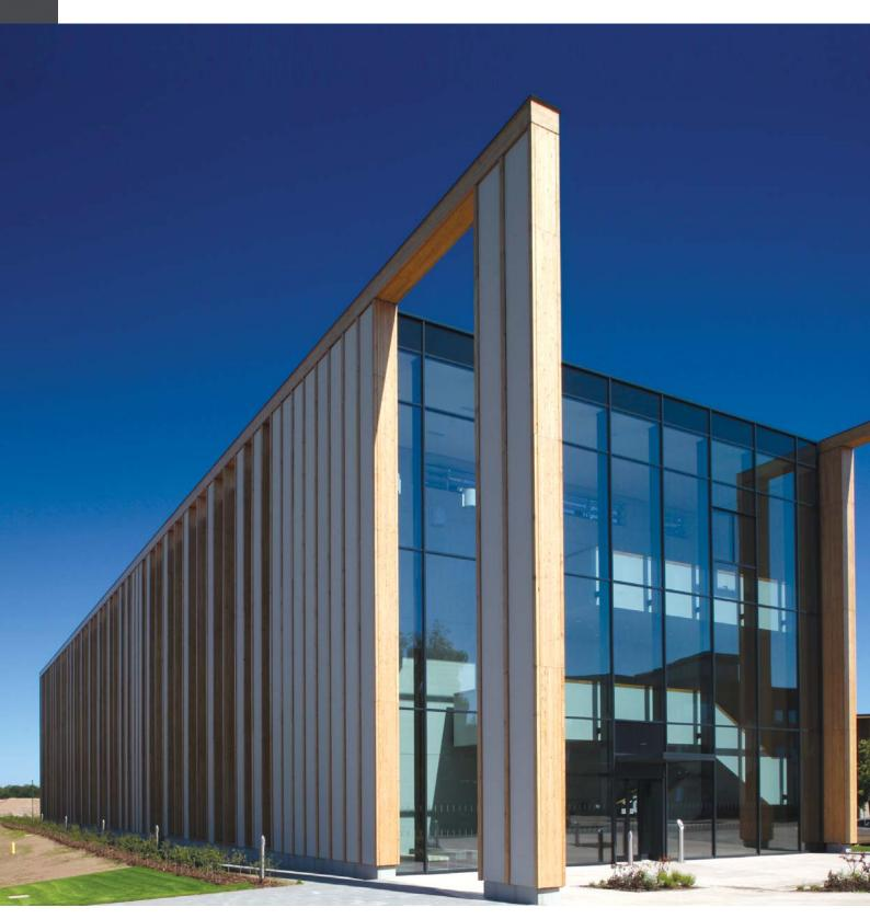
The SMR800 curtain wall system has been designed with enhanced thermal performance and to meet current building regulations. It is a stick system, zone drained and pressure equalized and offers a 50mm sightline, with a standard choice of six mullion and six transom depths. The system is designed for quick assembly on site and to accept glazing up to 28mm thick, depending on weight. Project specific profiles can be incorporated offering flexibility of facade design.
